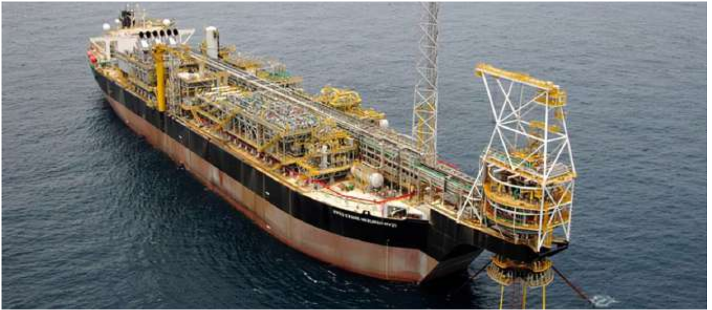
Figure 2: FPSO Kwame Nkrumah for the Greater Jubilee Field
